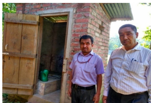
Toilet at Kangmong Tongbram Leikai with half brick masonry walls under Imphal West ZP
