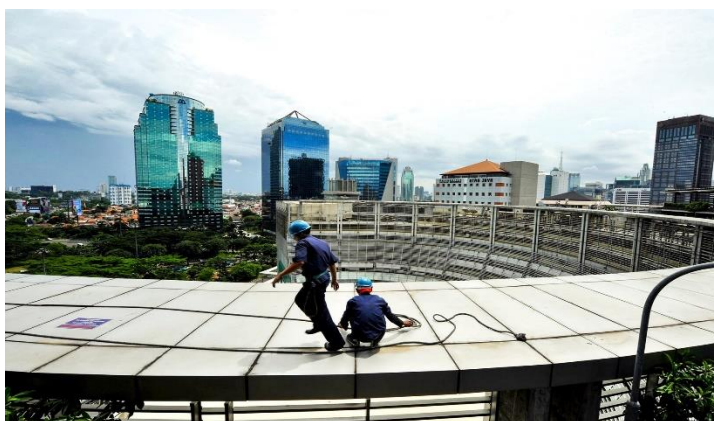
Two workers maintain installations on a skyscraper in Jakarta, Indonesia.
